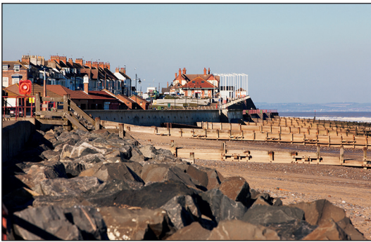
Figure 9a: Coastal protection, Hornsea, Yorkshire
